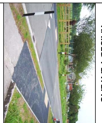
Normally full width of the road with a minimum 6 metre flat top to cater for easier movement of long vehicles, with a height of 75mm (subject to the tolerances permitted in the Road Hump Regulations, where the hump will not exceed 100mm in maximum height)
