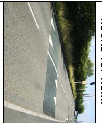
Tapered humps (humps that are not completely kerb-to-kerb) with a curved top surface. Minimum length 3.7 metres with a height of 75mm (subject to the tolerances permitted in the Road Hump Regulations, where the hump will not exceed 100mm in maximum height)
